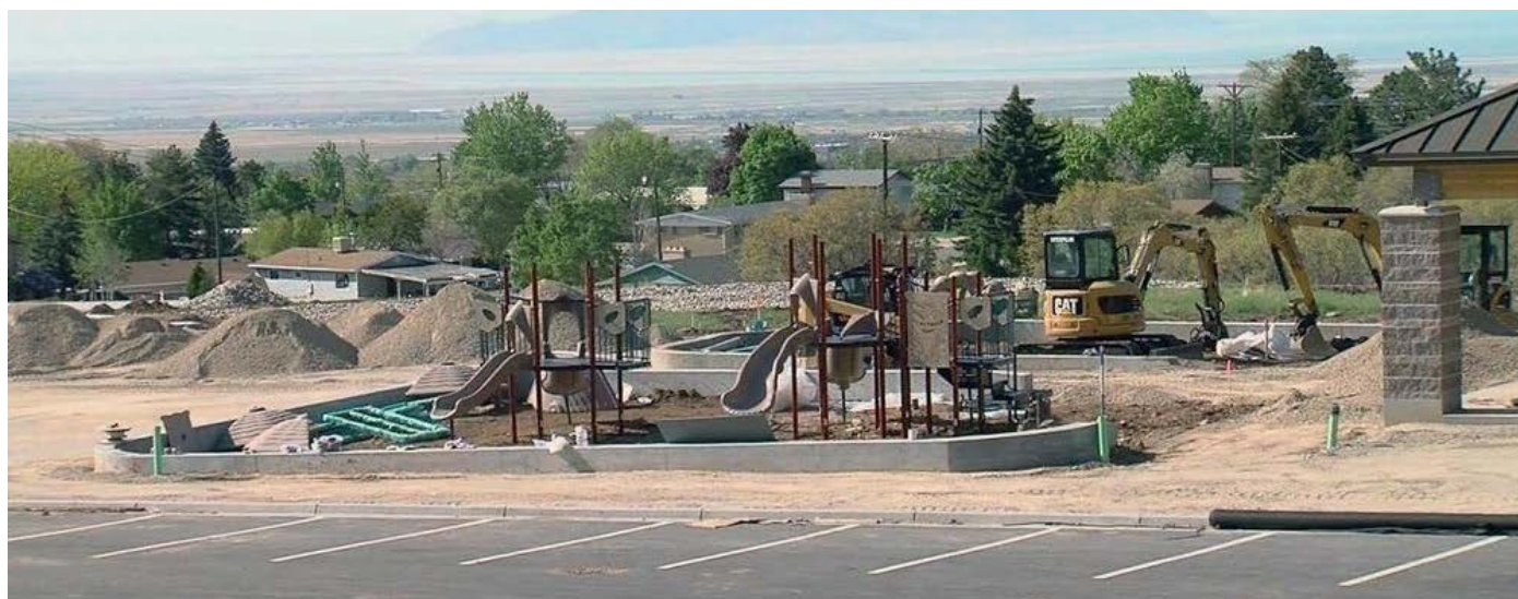
FIGURE 5: Construction of Skyline Nature Park
