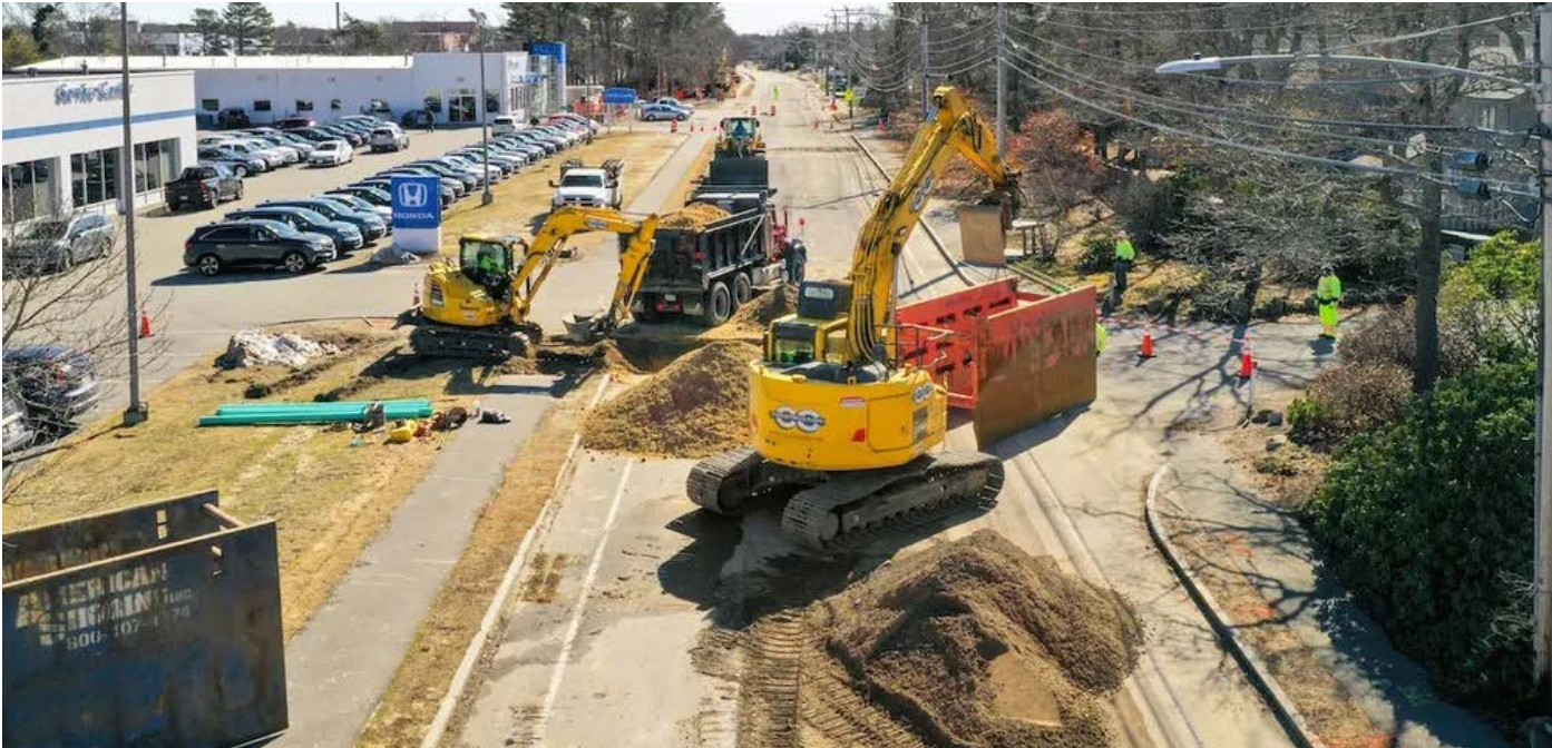
FIGURE 7: Sewer Construction Along Route of Vineyard Wind Cables
