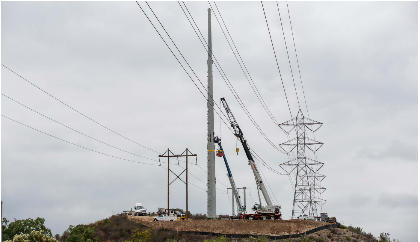
FIGURE 9: Sycamore-Peñasquitos Transmission Line Construction
