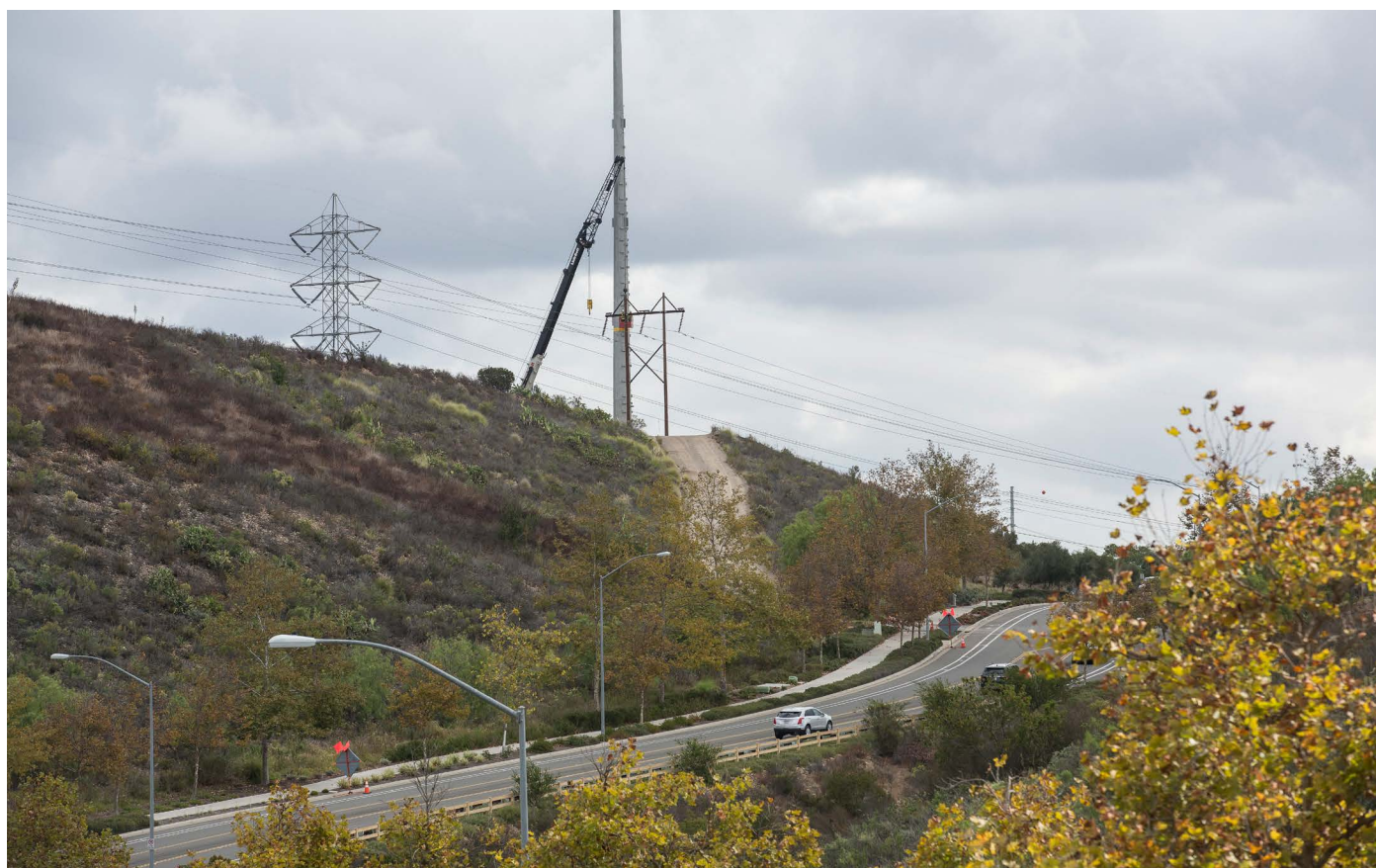
FIGURE 10: Sycamore-Peñasquitos Transmission Line Construction
