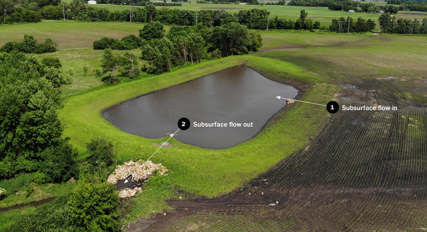
Figure 11: An active subsurface storage basin.
