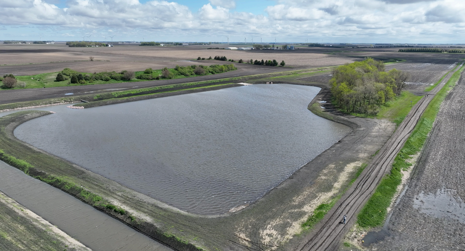
Figure 10: An active surface water storage basin.
