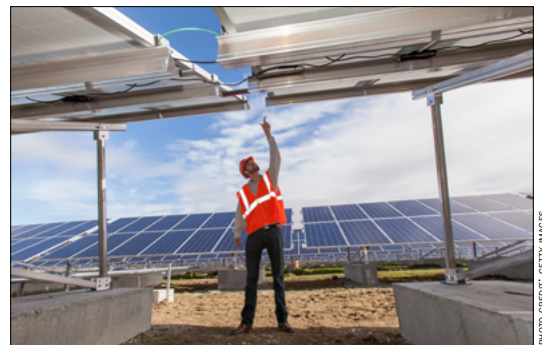
Solar photovoltaic installer examining racking for a PV array.
