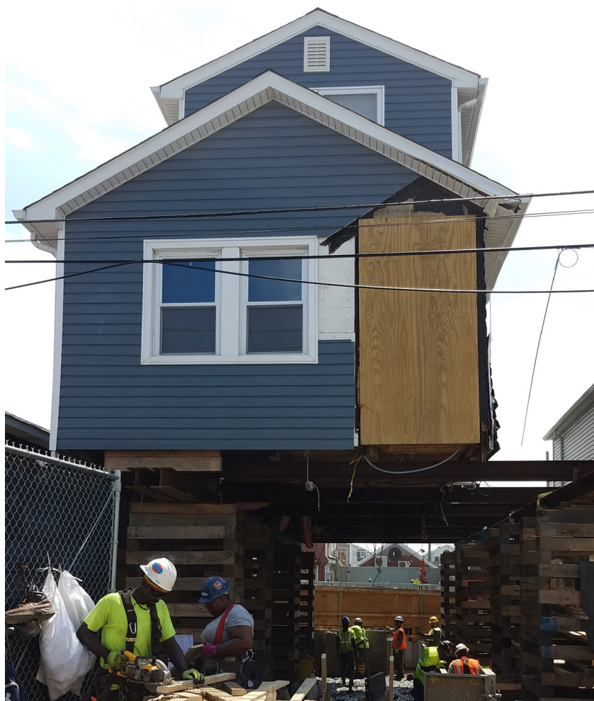
Home elevation work underway in Brooklyn to make it more flood resilient. Photo credit: NYC Mayor's Office of Housing Recovery Operations.
