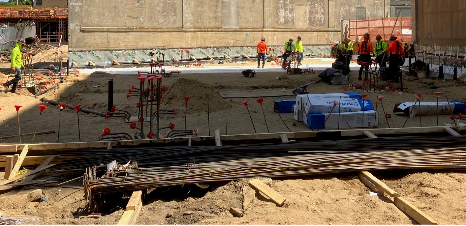
Construction of resilient housing in the Rockaways.
