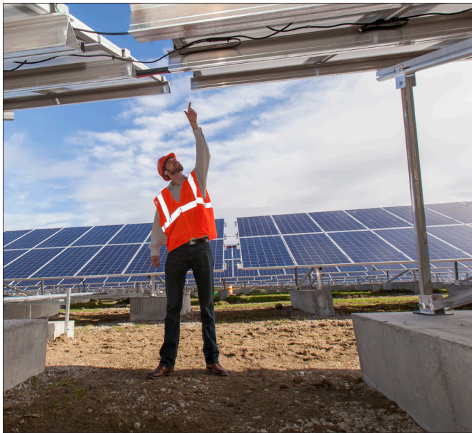
Solar photovoltaic installer examining racking for a PV array.
