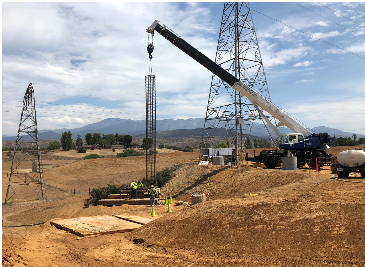
FIGURE 6: West of Devers Construction
